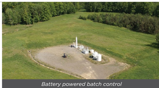
Battery powered batch control
