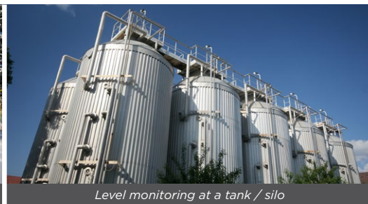
Level monitoring at a tank / silo
