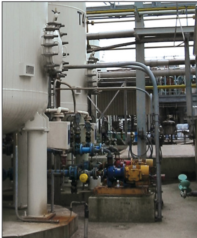
Figure 1: FCI Model FLT93S flow/level switch protects pumps from dry-running and other operational downtime conditions
