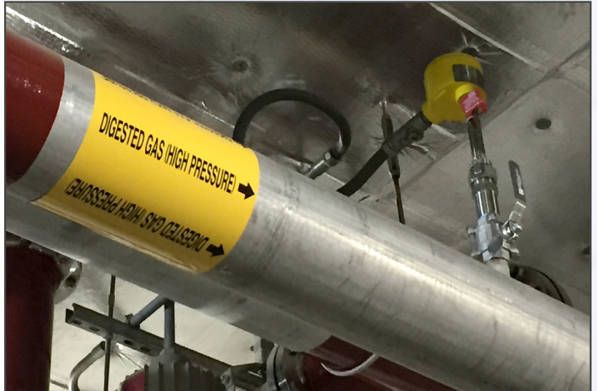
Figure 1: Knowing gas type is required to specify a thermal flow meter
